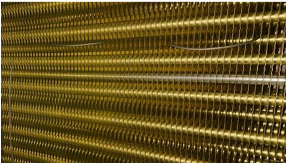
Here is the correct wiring shown on a direct expansion evaporator. The wire is going through the evaporator.
