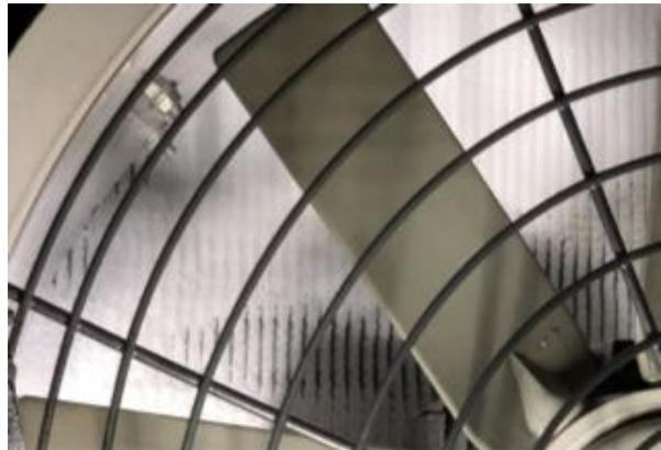
Air outlet side on the same evaporator covered blocked with ice
