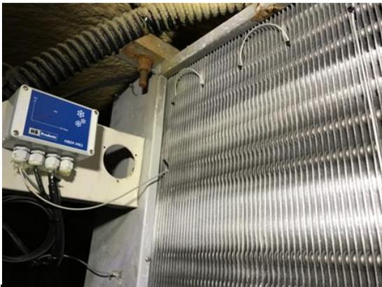
Air inlet side with limited ice due to superheat.
