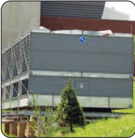
An evaporative heat rejection device enables building owners and operators to take advantage of the operating cost savings inherent in water-cooled systems. A well-maintained tower enables the entire cooling system to perform at optimum efficiency by conserving both energy and water.
